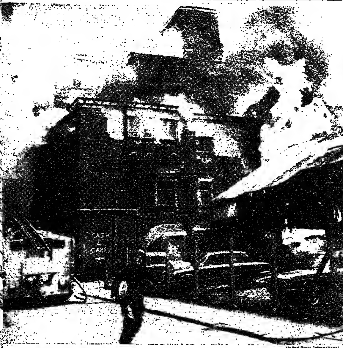
destroys a building in Belfast after seven bombs exploded in an hour at five targets in the city
